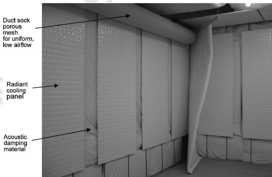
55 Fig. 5. Photograph of the STEM room at Bell Labs circa 2002. Fiberglass acoustic banners are hung ~6 in off the wall and behind the radiant cooling
